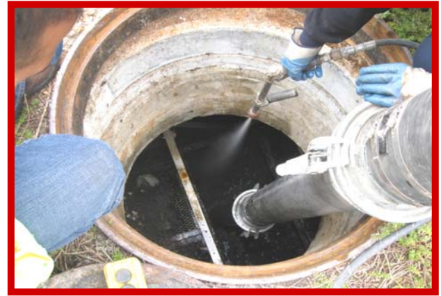
Insert Vacuum Hose in the Sedimentation Chamber and Vacuum Out All Trash, Sediment and Standing Water.
