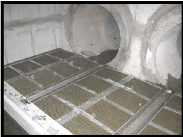
Assess the Condition of the Media in the Up Flow Filter. Remove Old Media When Necessary.
