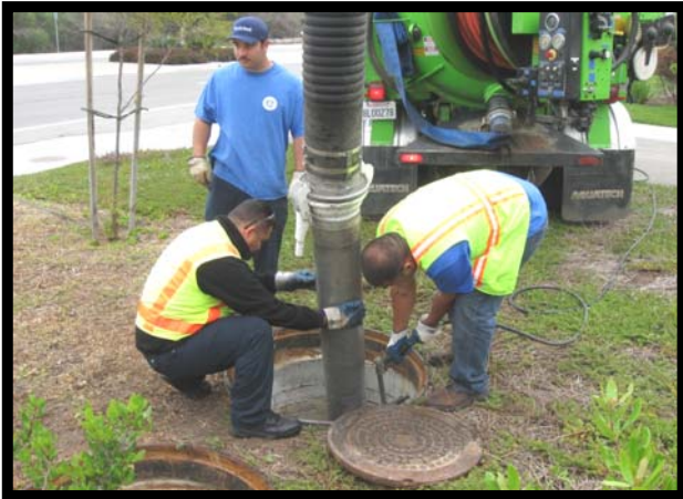
Remove Access Hatches and Inspect Sediment Accumulation in the First Chamber.
