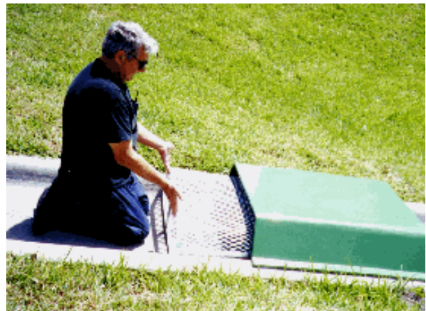
STEP 4: Replace Filtration Chamber
