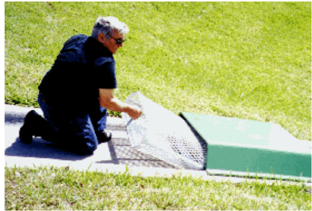
STEP 2: Pull out Filtration Chamber
